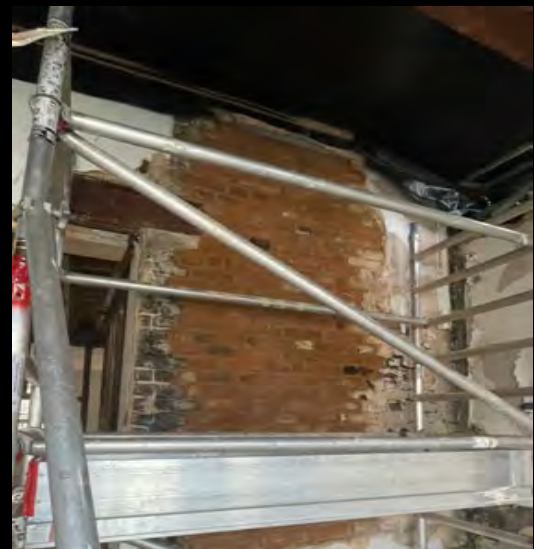
Heritage brickwork repair in 16 SMS
