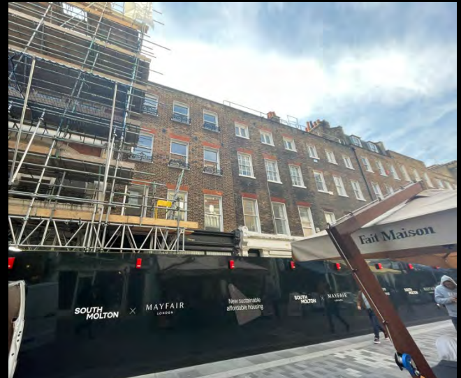
Scaffold erection continues behind the hoarding at SMS
