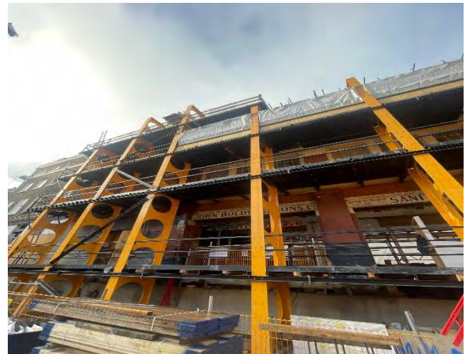
Our new façade retention structure.
